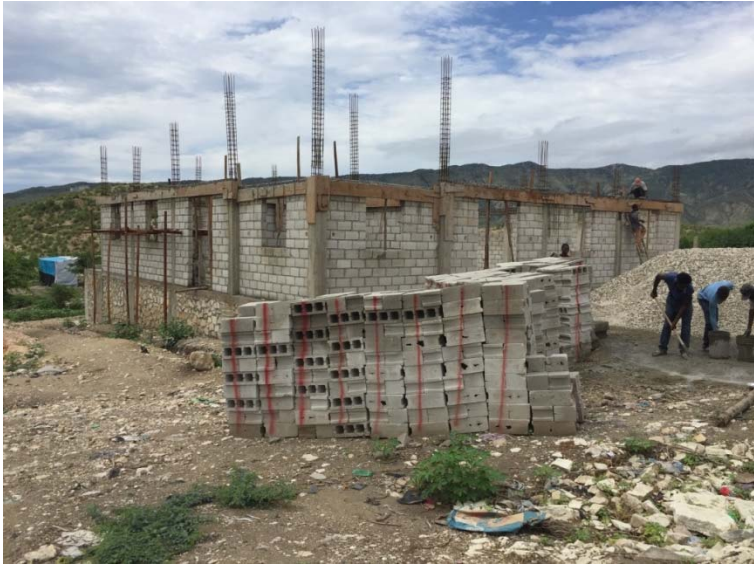
Construction of The Truth Presbyterian Church.
